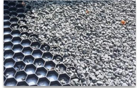
Figure 11.10-15: Example of permeable paving surfaces (guideline 6g)
