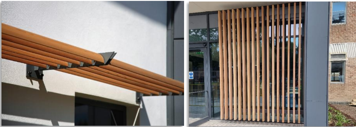
Figure 11.10-11: Examples of solar shading on south facing windows (guideline 4a iii)
