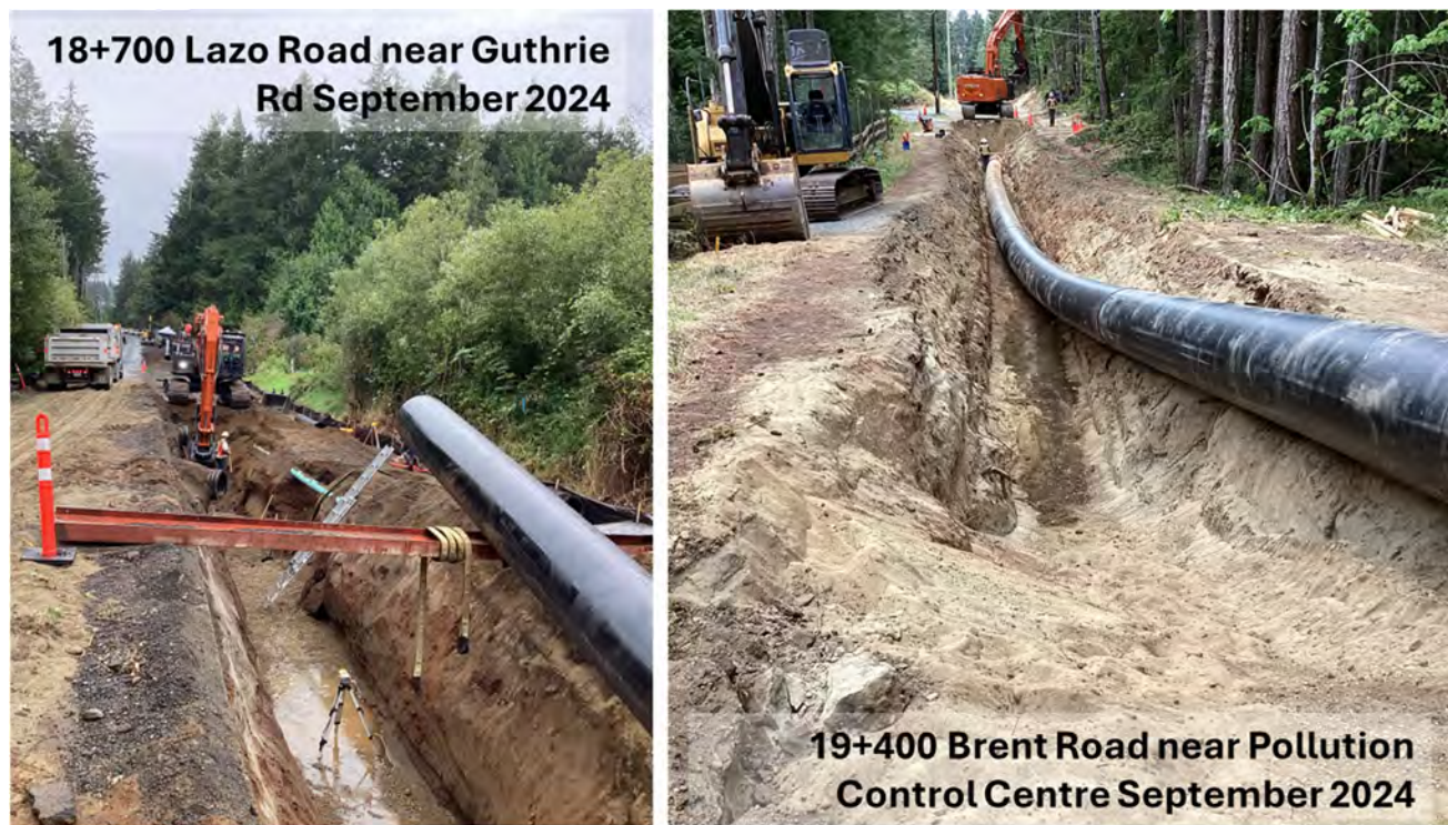
Figure 5: Example photos of trench and pipe installation. Photos from CVRD.
