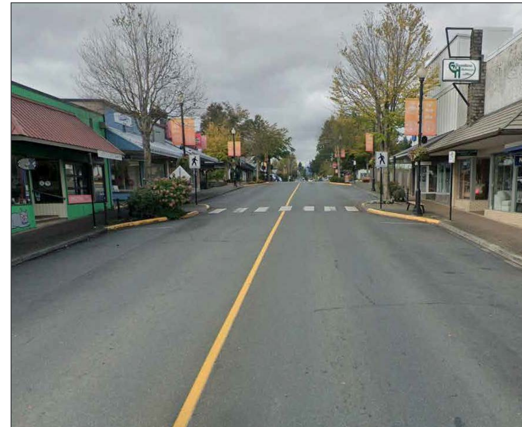
5th St Existing Conditions
